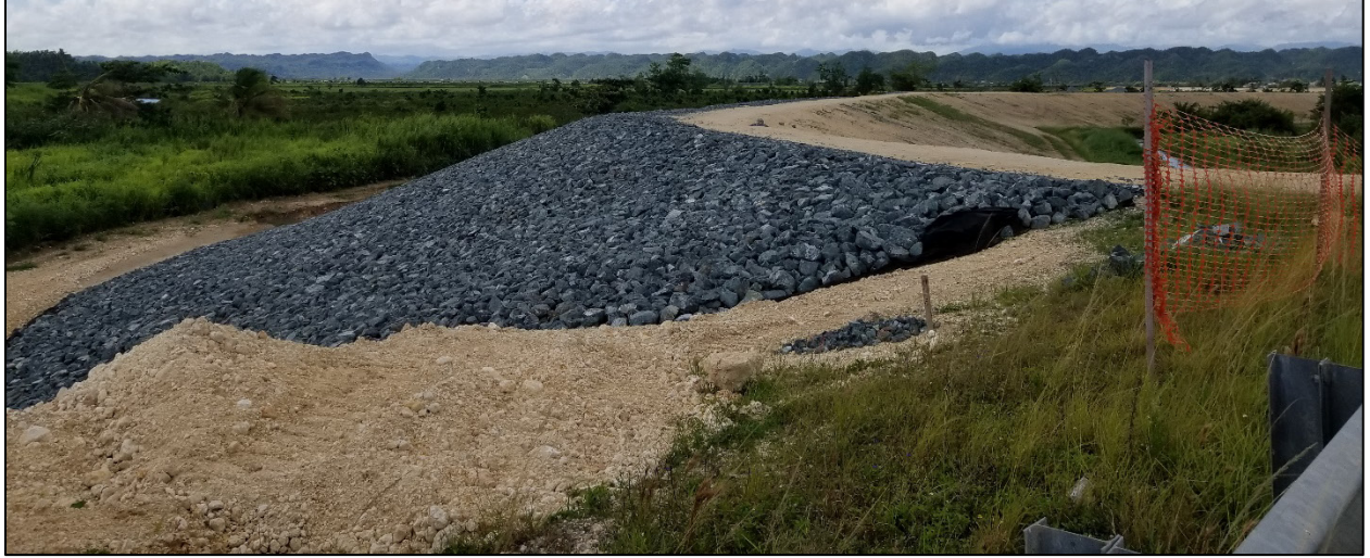
Figure 4-8: Road Elevated Above Flood Line in a Flood Zone
