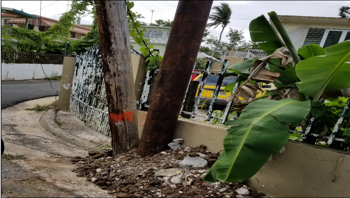
Figure 4-14: Electrical Grid Repairs
