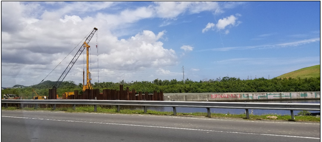
Figure 4-10: Piles Driven into the Ground for Bridge Reconstruction
