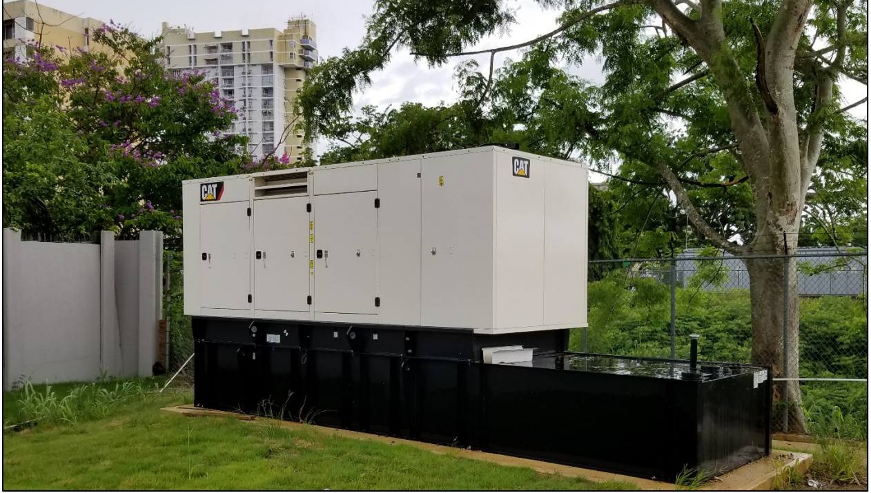
Figure 4-16: Generator Being Installed in a Mixed Use Development
