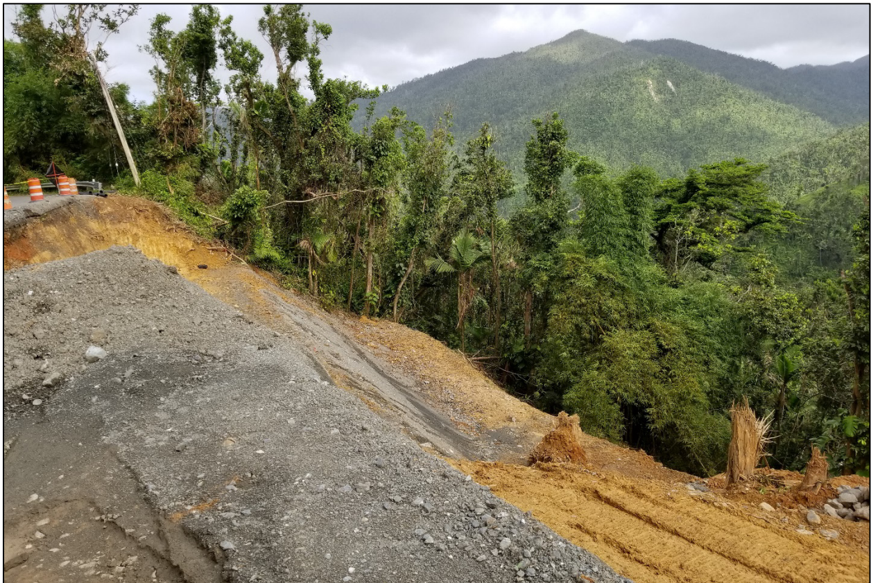
Figure 4-3: Las Piedras Landslide Repair in El Yunque
