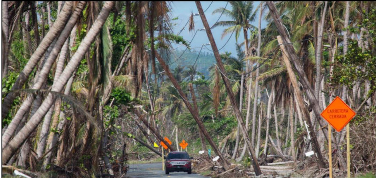
Figure 2-1: Example of Downed Power Lines in Puerto Rico (Image Courtesy GAO, 2019)
